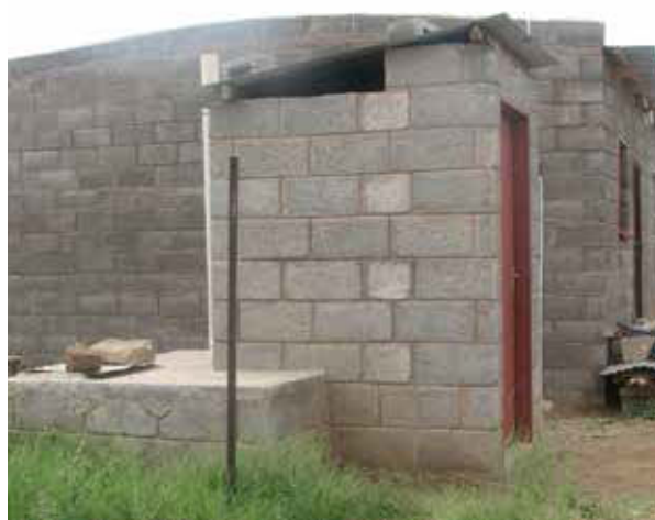
FIGURE 62 VIP toilet showing vault at the rear. Most ventilation pipes are white instead of the recommended black so that they would be hot.
