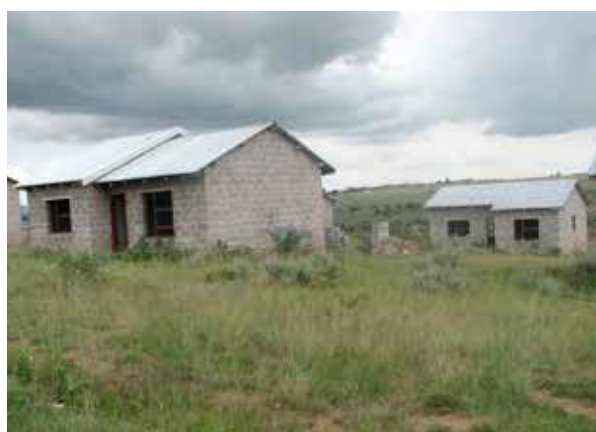
FIGURE 83 Complete experimental Hydraform block dwelling built by MLGCPA
