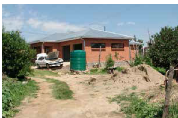
FIGURE 60 Water tank for roof run-off
