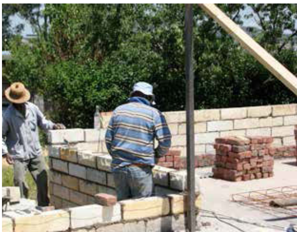
FIGURE 73 Informal construction using high quality materials; machine cut stone and local bricks
