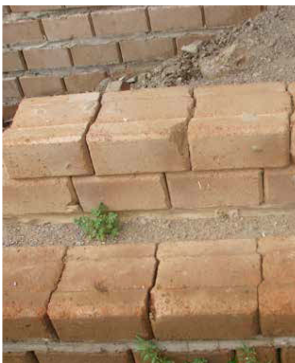
FIGURE 85 Corner and base detail of hydraform under construction
